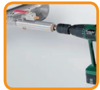
Drilling under pressure
